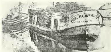
Canal boat loaded with fire wood for trip between New Haven and Fort Wayne, last used portion of the canal in this area.
